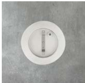
1. The pot is cast into the concrete of the pool wall.
