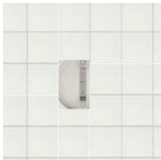
2. Tile partially over the recessed housing.
