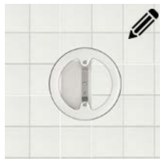
4. Mark the mounting ring with a marker.
